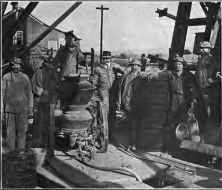
APPARATUS SET UP FOR WORK AT COLLAR OF "A" SHAFT
